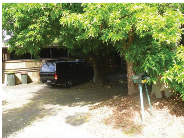
13. 126A Epping road (facing southwest)
