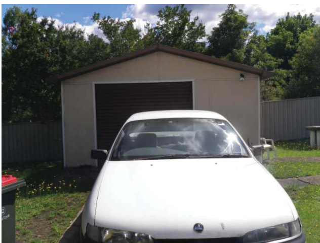
9. Garage/Shed located at 366 Lane Cove Rd – fibro sheeting, possible asbestos containing material.
