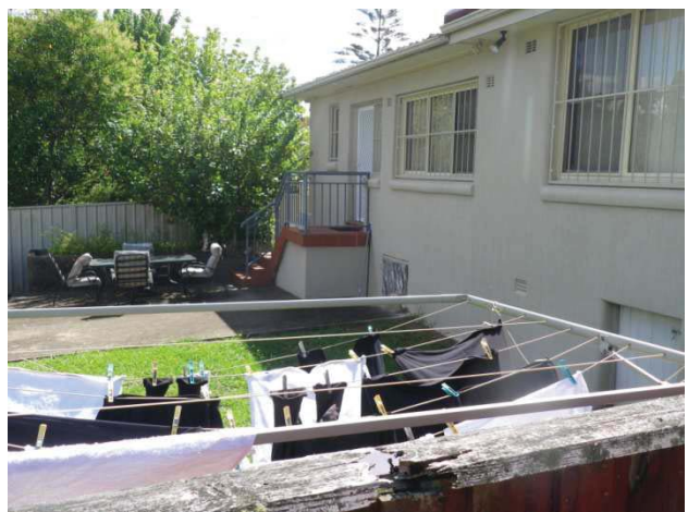
10. Crawl space identified at 366 Lane Cove Rd
