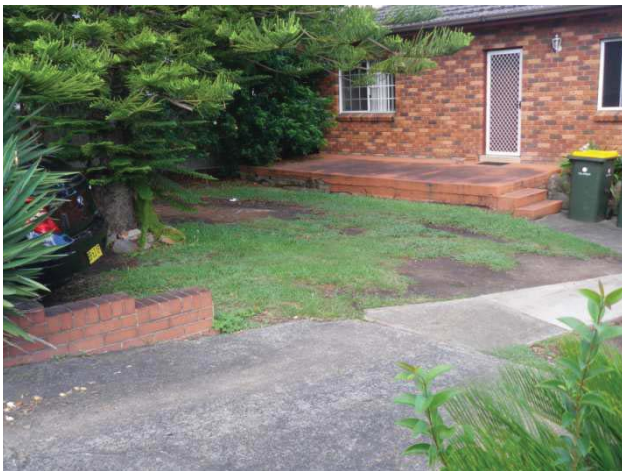
7. General soil erosion, 372 Lane Cover Rd (facing west).
